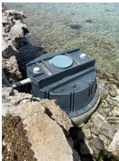
Image 22 – Old sewage outfall pipe. Image 23 – Approved septic tank system.
